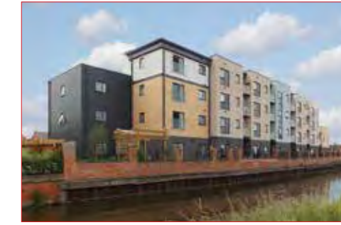
Waterside Court, Loughborough submitted by brp architects
