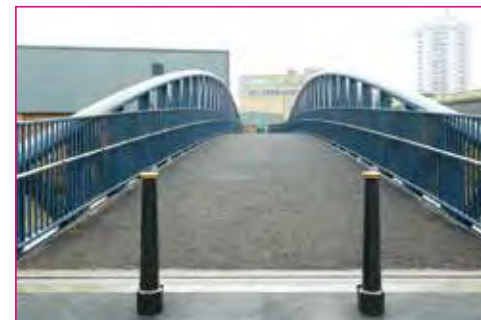
Charter Street Footbridge, Leicester submitted by Danaher & Walsh and Leicester City Council
